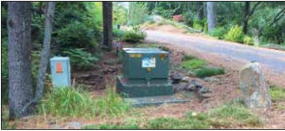
Change in elevation: The transformer on page 1—after we added a ground structure to keep it above water following heavy rains.
