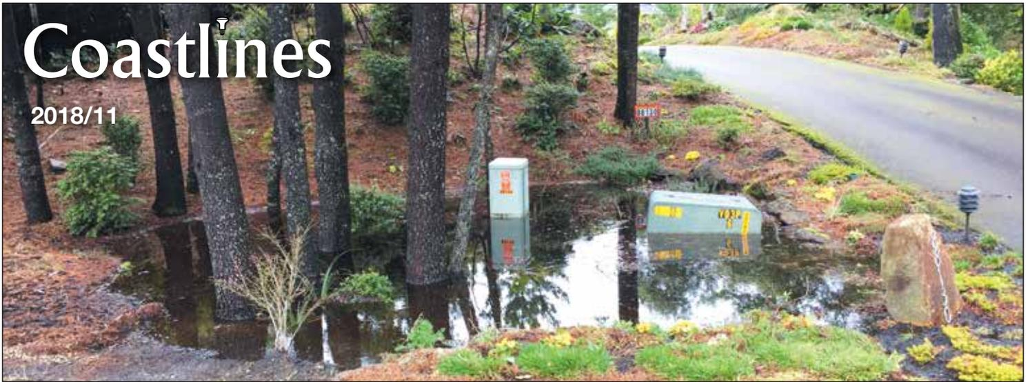
*A sharp-eyed customer spotted this submerged pad-mounted transformer, and called us. We were able to move it above the water line. Transformers should not be touched. Why? See page 2.*
