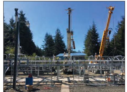
A crane and two trucks were required to lift the 15,000 pound ground-level assembly 15 feet in the air for final touches.
