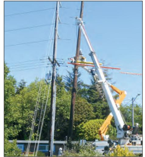
*One of the biggest 'needles' ever? Linemen carefully position a new power pole to replace an aging one while the attached lines are still energized.*
