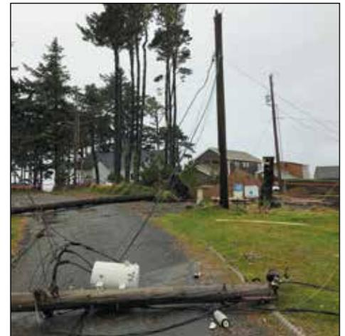
A squall during the Thanksgiving weekend last year slammed a tree down on power lines with such velocity a utility pole snapped.
