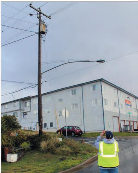
*Distribution Technician Brandy checks out an overloaded transformer she will soon have replaced by a line crew. Power distribution transformers transform power from higher voltages used for distributing electricity over distances, to voltages suited to residential, commercial, or industrial uses.*
