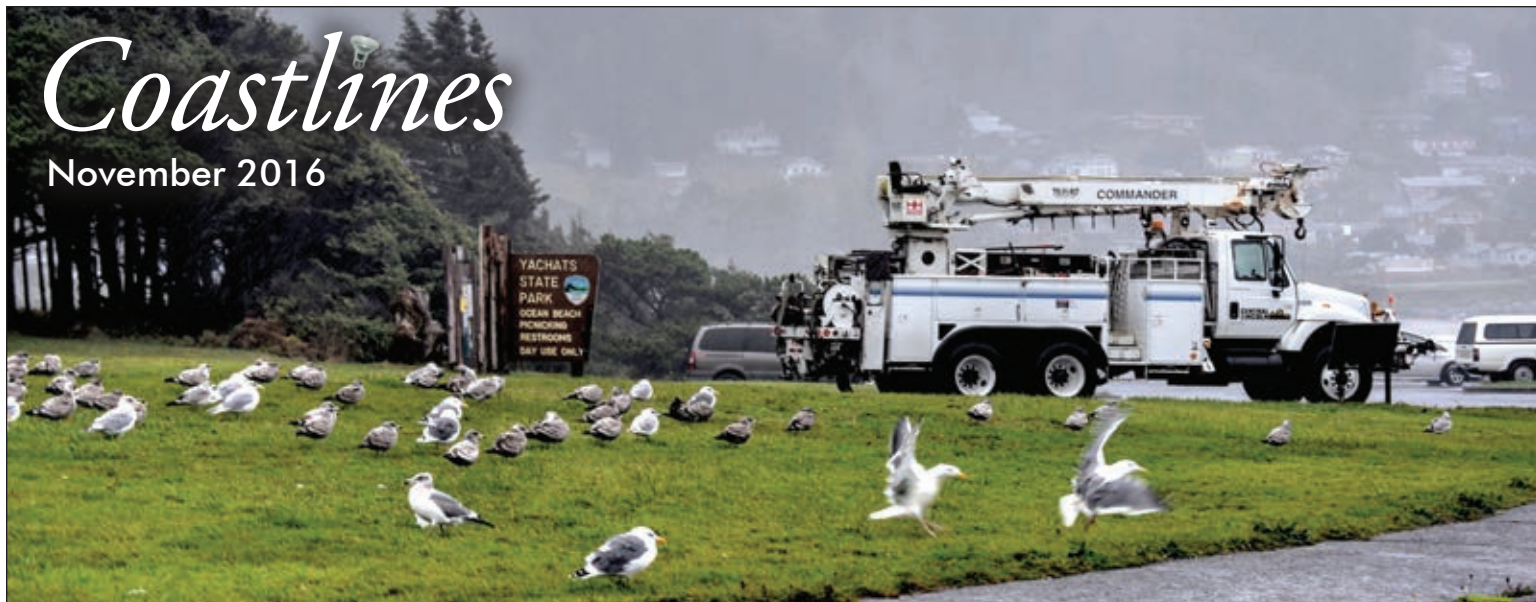
Seagulls surround a Central Lincoln "digger derrick" truck during a brief lunch break between storm squalls Photo © Ken Gagne
