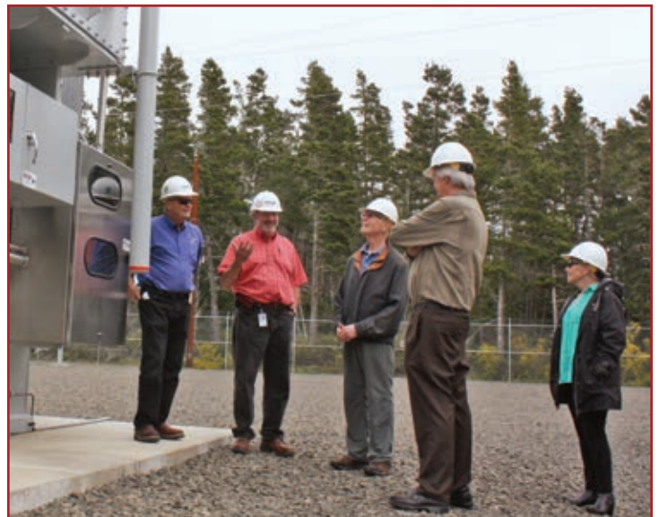
Reviewing results: Board members get a firsthand look at Central Lincoln’s new substation in the Pacific View Business Park in Florence with (left to right) Engineering Manager Bruce Lovelin and Senior Systems Engineer Steve Alexanderson. Listening to Lovelin and Alexanderson’s presentation are Board Members Larkin Kaliher, Curt Abbott and Judy Matheny. (Not shown: Board Members Ron Benfield and Tom Tymchuk.)
