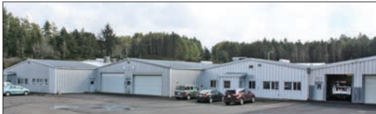
Our substation, communications, and meter operations serve our entire District from this facility in the South Beach neighborhood of Newport. Unfortunately, this location, which was built after World War II, is in the tsunami inundation zone.
